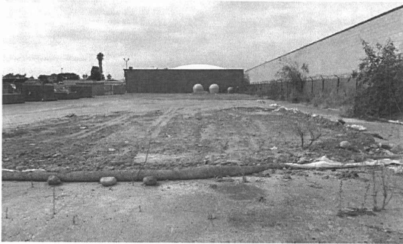
Figure 4: Soil, Asphalt & Gravel to be Removed
