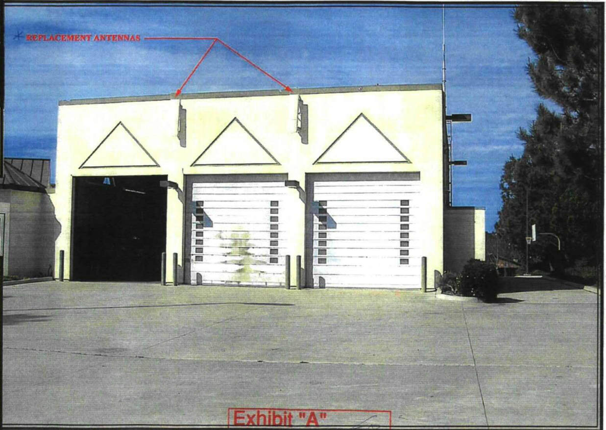
SITE AFTER INSTALLATION
