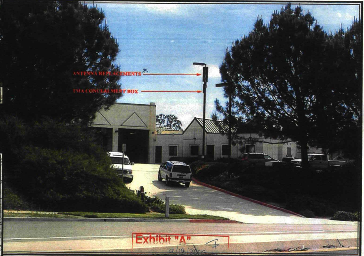
SITE AFTER INSTALLATION
