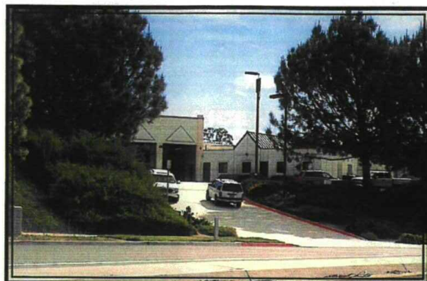
SITE PRIOR TO INSTALLATION
