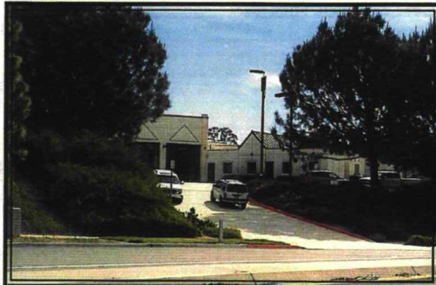
SITE PRIOR TO INSTALLATION
