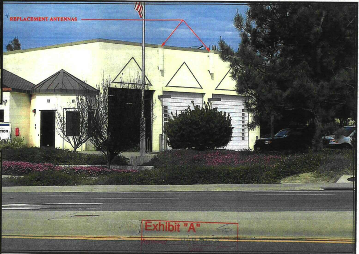
SITE AFTER INSTALLATION
