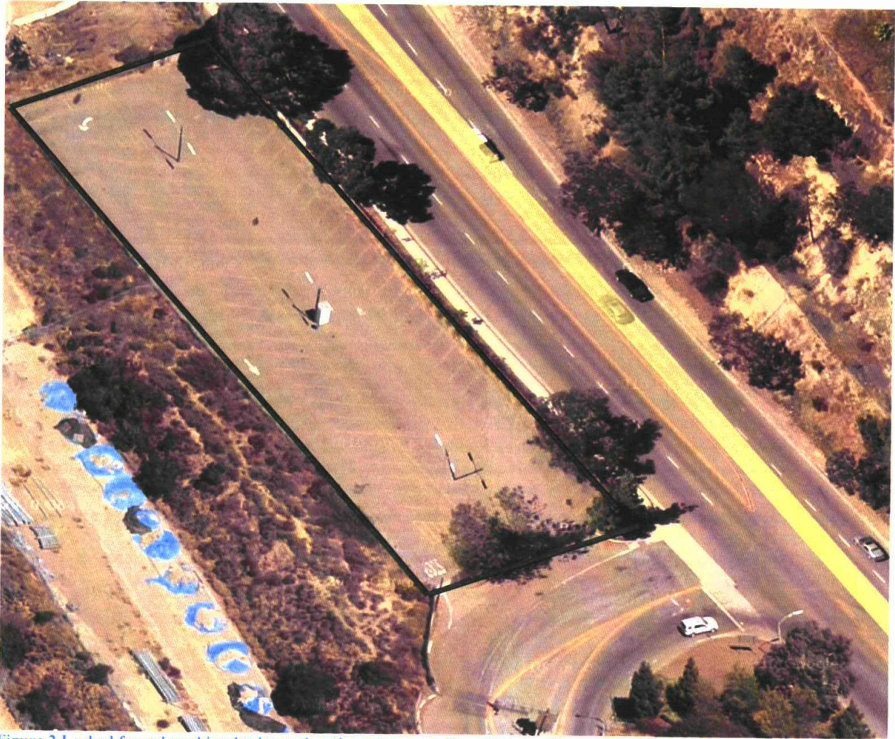
Figure 2 Locked fenced parking lot located at the entrance to Rose Canyon Operations Center (Storage of light equipment, construction vehicles, pvc pipe, vaults and pedestals)
