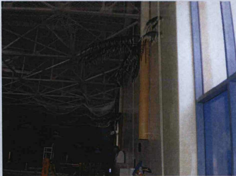
Figure 10. Furnace Air Ducts Painted as Palm Trees
