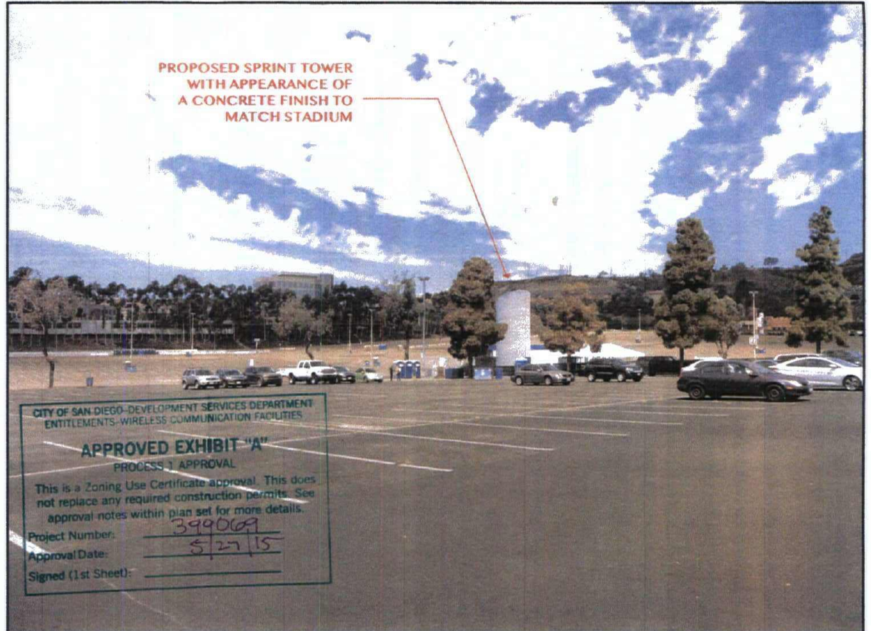
SITE AFTER INSTALLATION
