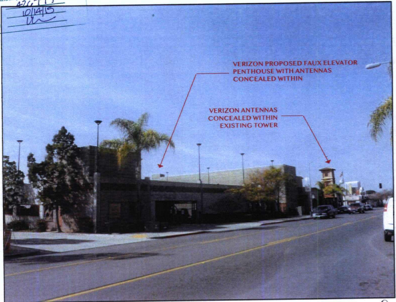
SITE AFTER INSTALLATION
