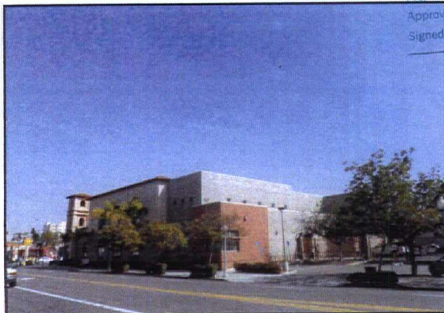
SITE PRIOR TO INSTALLATION
