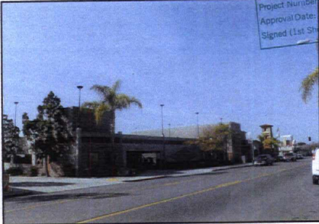
SITE PRIOR TO INSTALLATION
