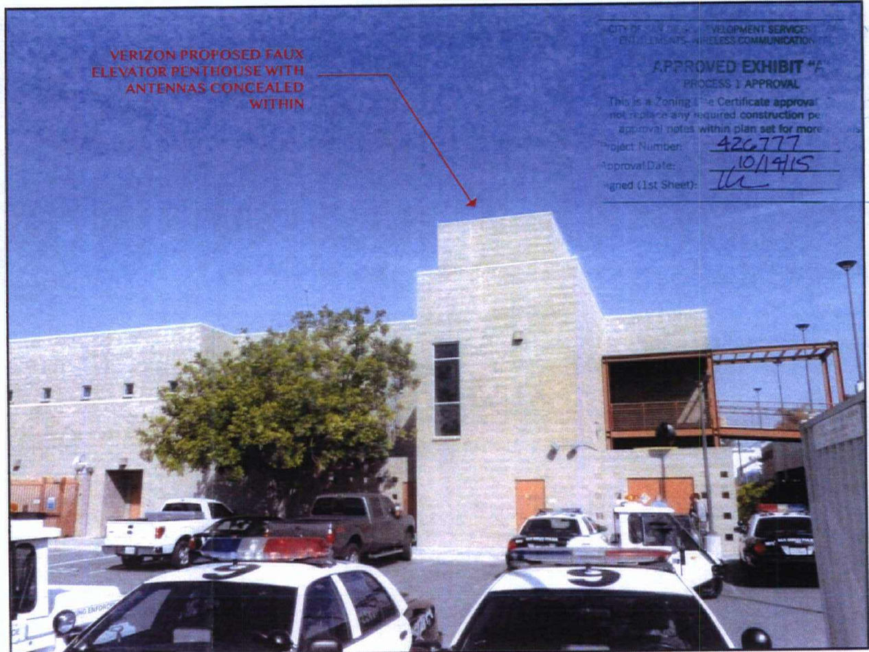
SITE AFTER INSTALLATION
