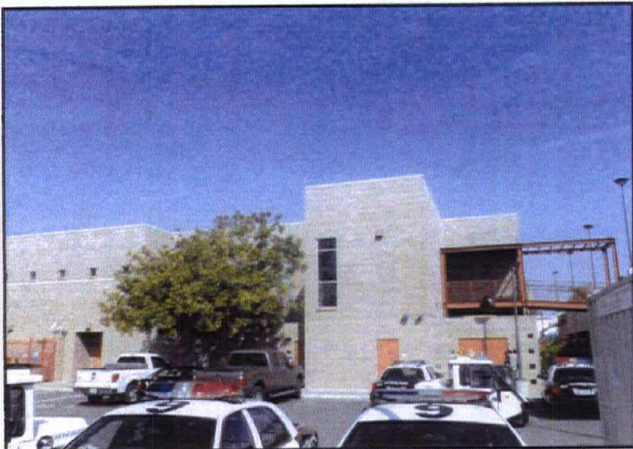
SITE PRIOR TO INSTALLATION
