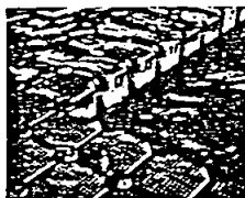
The fingerdocks are securely interlocked with the main dock and form one sturdy floating structure of great stability.
