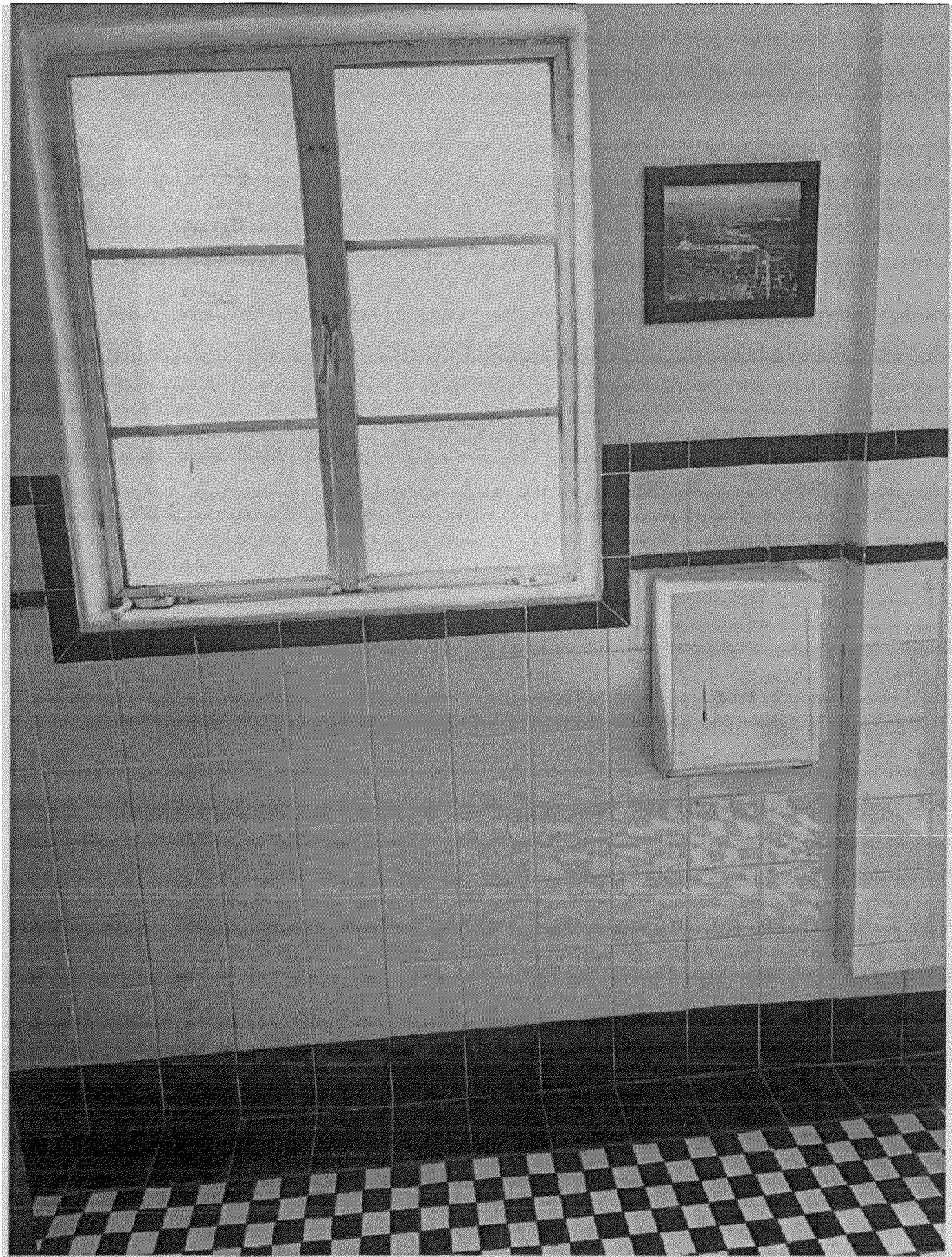
Single paned window. Will be replaced with dual paned energy efficient window.
