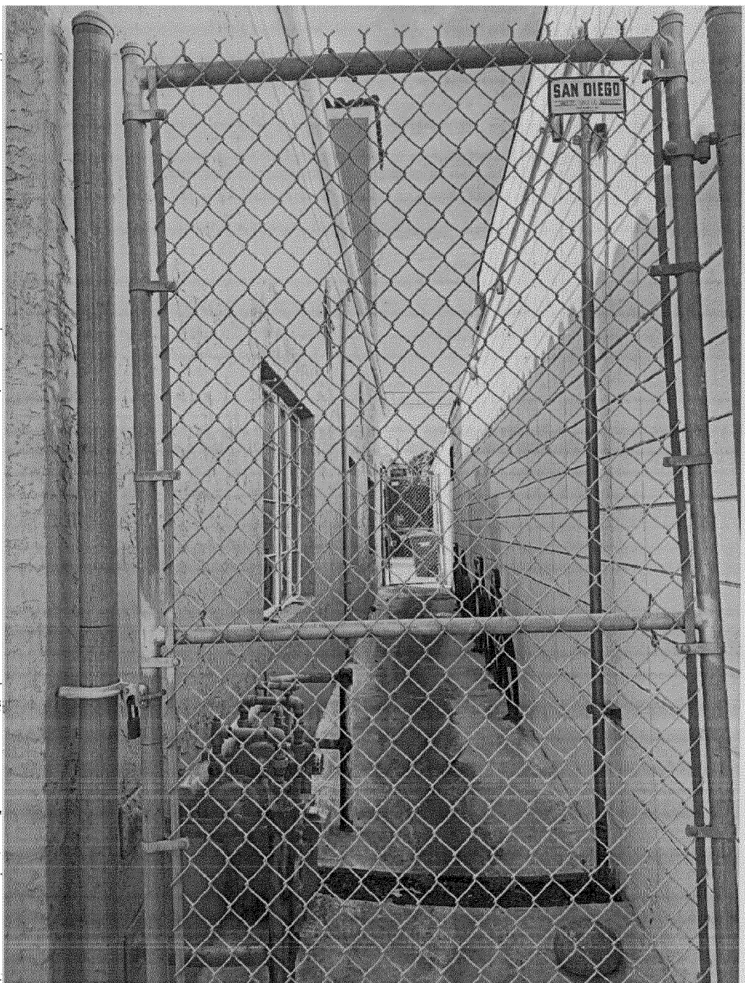
Interior locked and fenced path between buildings. Utility meters. First floor casement window.
