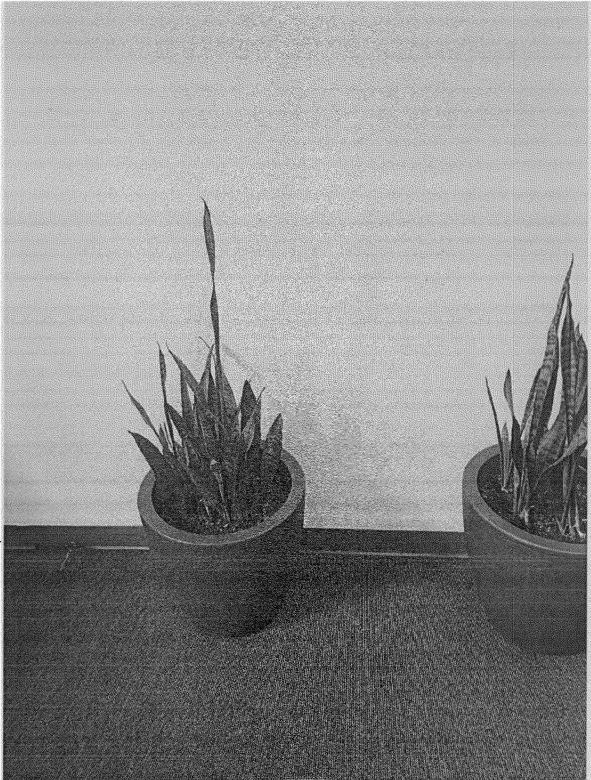
Frayed carpeting. Will be replaced.
