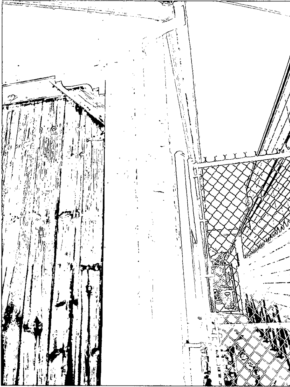
- Exposed wood on shed.
