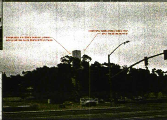
SITE AFTER INSTALLATION
