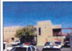
SITE PRIOR TO INSTALLATION
