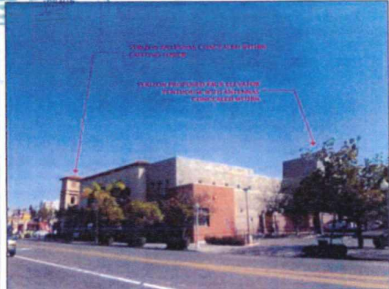
SITE AFTER INSTALLATION
