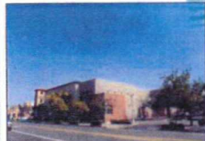
SITE PRIOR TO INSTALLATION
