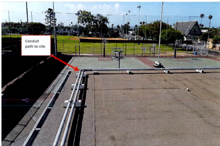
1 B-2 PHOTO: FIBER PATH NOT TO SCALE
