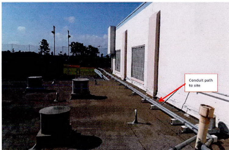
3 B-2 PHOTO: FIBER PATH NOT TO SCALE
