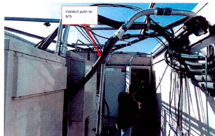
4 PHOTO: FIBER PATH TO BTS CABINET
