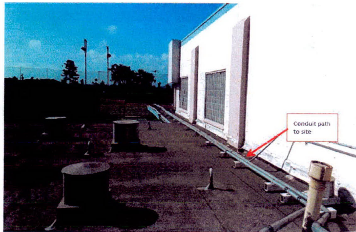
3 B-2 PHOTO: FIBER PATH NOT TO SCALE
