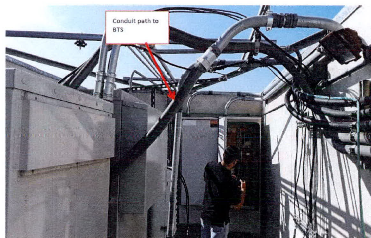
4 PHOTO: FIBER PATH TO BTS CABINET
