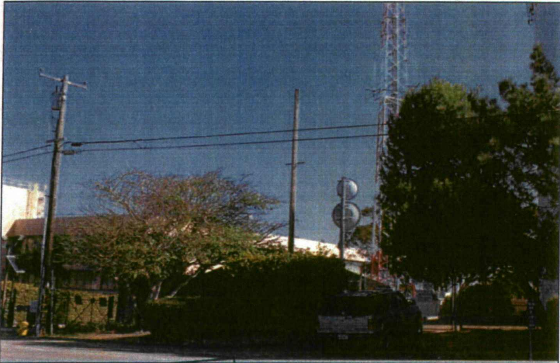
VIEW #3 - Looking EAST from Catalina Blvd at existing 60'-0" wood utility pole (center of photo). Verizon proposes to temporarily attach two (2) antennas stacked vertically to existing pole (30'-0" to top of proposed temporary antennas)
