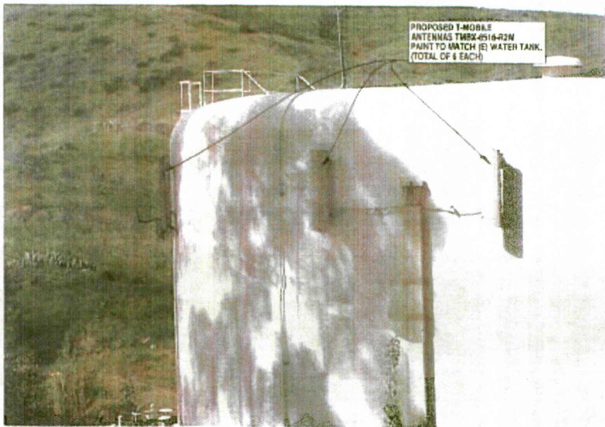
SITE AFTER INSTALLATION
