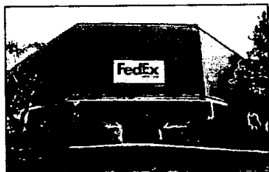
Kearny Villa Court (Industrial) Kearny Mesa 90,038 SF
