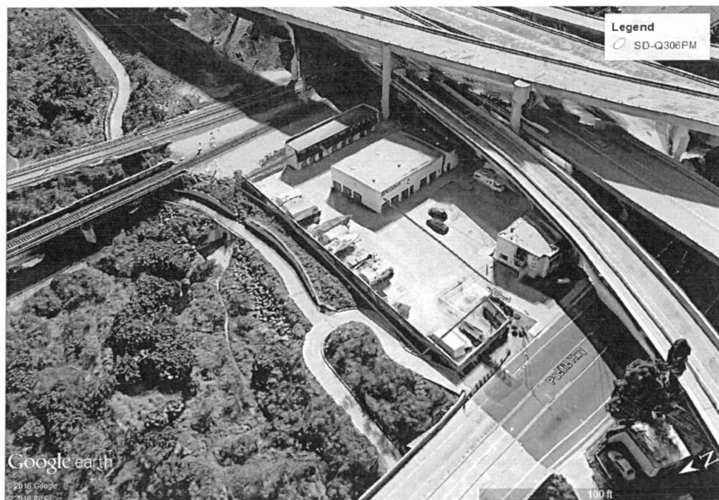
The property boundaries are approximate. The two encroaching buildings are indicated in the photograph.
